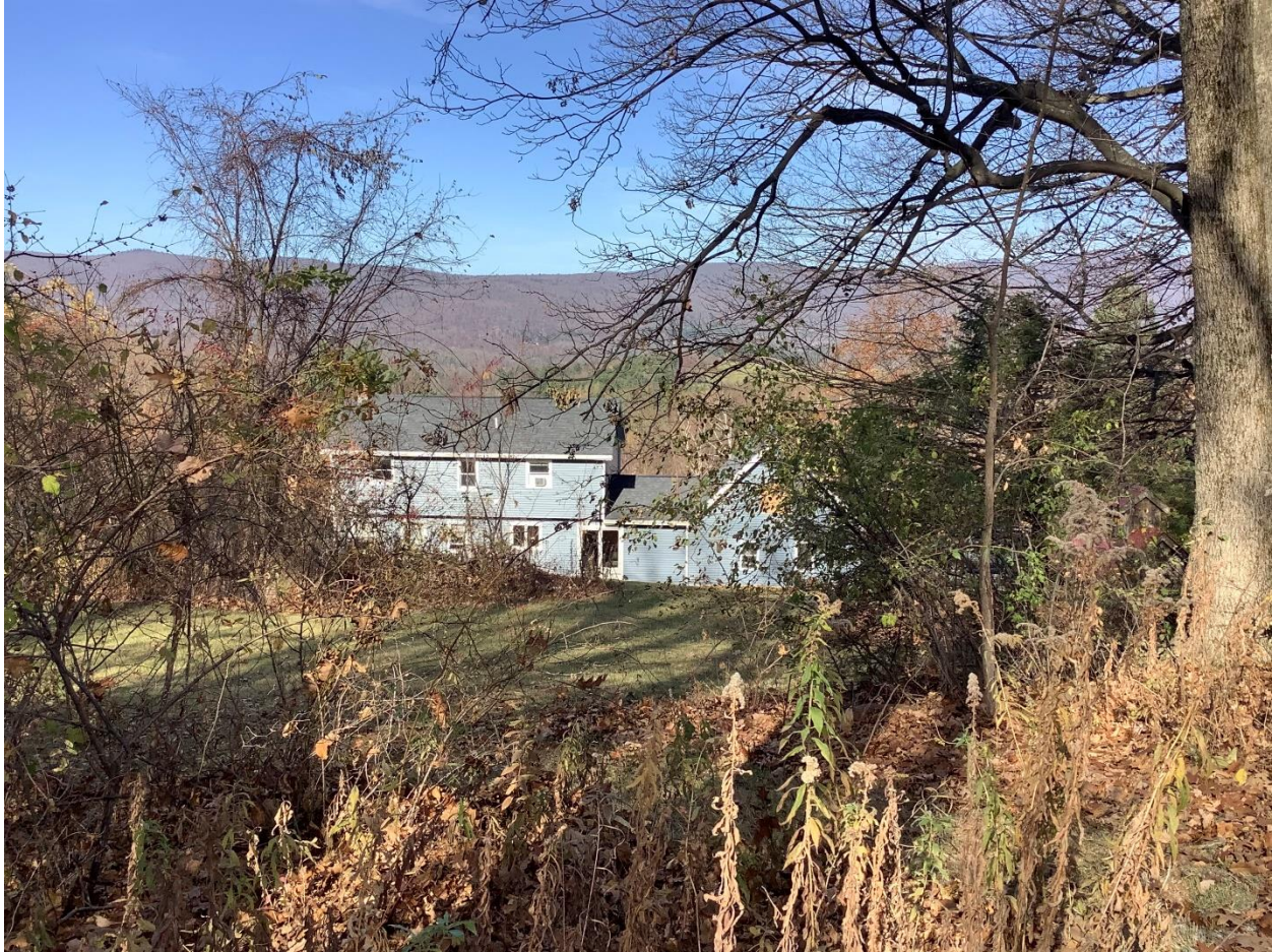
Photograph 13: Looking northwest at 708 Holy Smoke Road (Map ID D) from the northernmost boundary of the Project site. 708 Holy Smoke Road was constructed in 1987.
