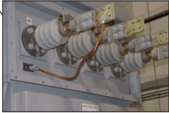
Side Mounted LV Bushings
